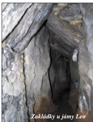
Štoly pod trati
